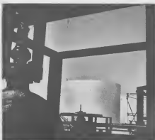
SUPPORT IN the form of I beams, common in the building trade, is needed to bear the weight of heavy steel plates for a round storage tank roof. AGUANTE DEN forma di balkinan den forma di I, común den construcion, ta necesario pa carga e peso di plachi di ataal piñá pa dak di un tanki rondó.
